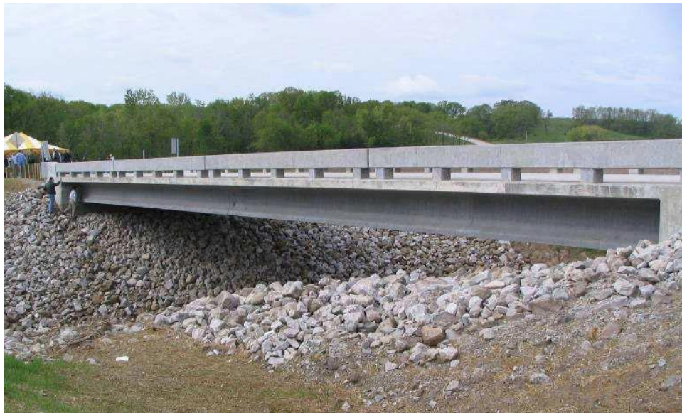
Figure 2.3: Mars Hill Bridge completed.
