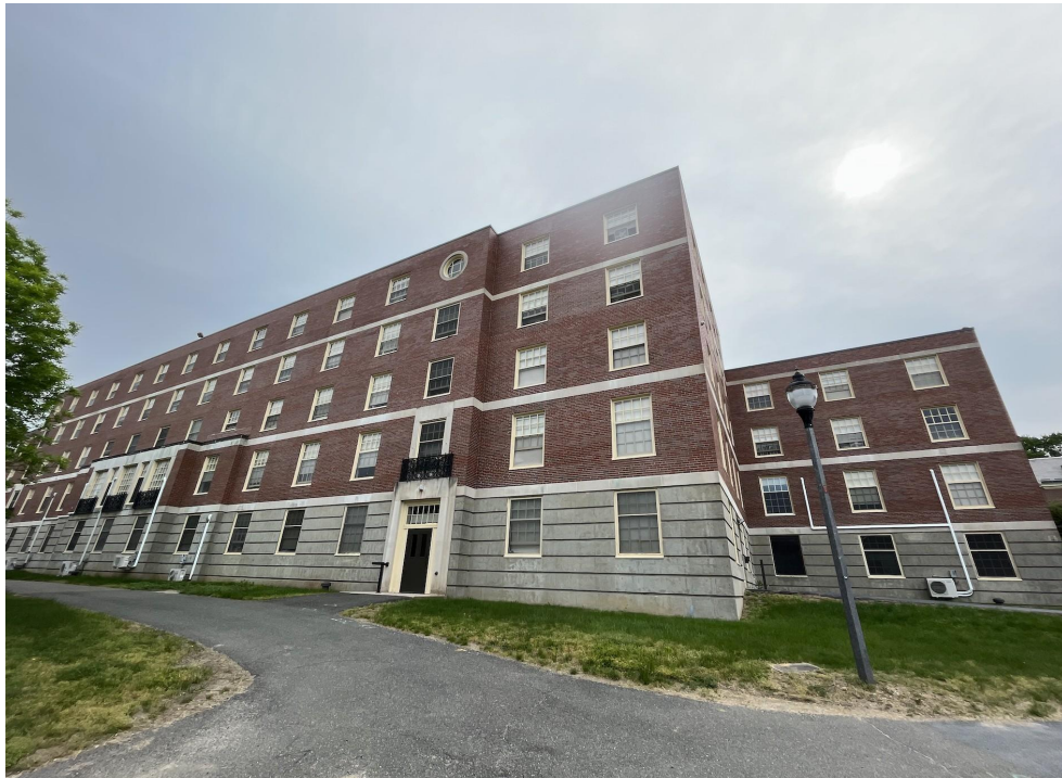
Figure 8: Brett Hall from Campus Side
