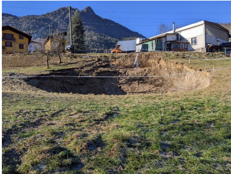
Figure 2: Sinkholes already present in the site
