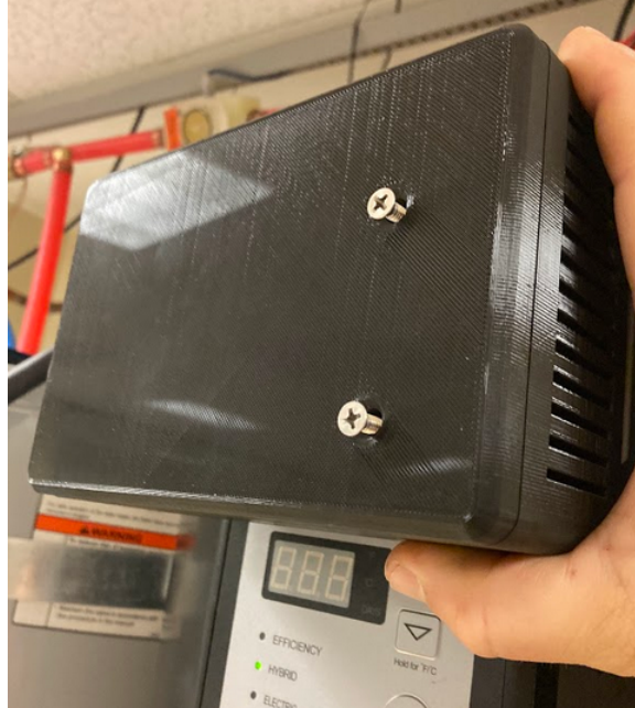
Figure B.6 Supporting the DCM by hand while installing mounting hardware
