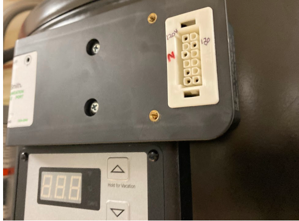
Figure B.2 Female 12 pin connection located on the adapter module
