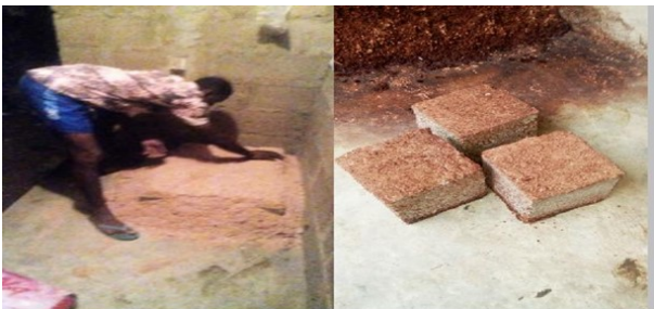
Figure 3. Wet Curing with Sawdust
