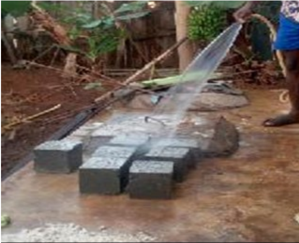
Figure 2. Water Sprinkling Curing
