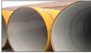
Fig 2: Cement coating of the inner wall of water steel pipeline
