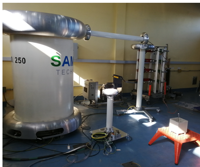
Figure 6. Step-up transformer and test cell for the AC dielectric strength tests.
