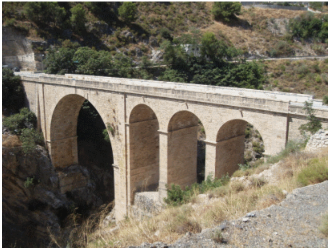
Figure 13: Izbor Bridge (Granada), with a 23-m-span main Arch and Three 7-m-span Access Arches, on the Primary Road from Granada to Motril. Third Quarter of the 19 th Century
