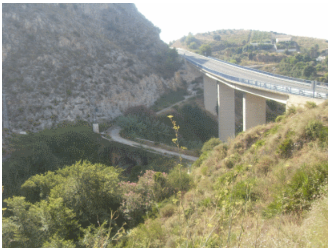
Figure 29: Bridge of Masonry Arches Near Nerja (Málaga), on an Abandoned Road from Malaga to Almería along the Coast. The Modern Bridge that Appears in the Background is on Another Old Stretch of the Highway, Today Replaced but Still in use as a Secondary Road
