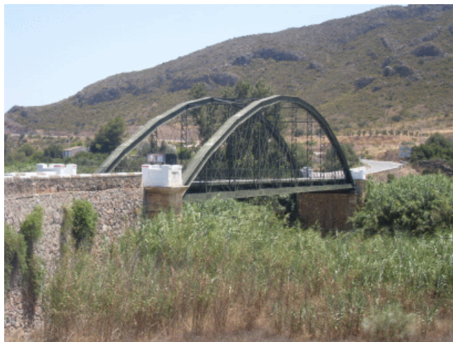
Figure 21: Bridge over the Almanzora River in Cantoria (Almería), with a Bowstring Arch having a 60-m Span, 1925. Ángel Ochotorena, Civil Engineer
