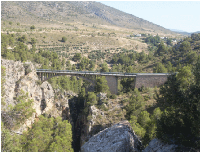
Figure 25: Bridge over the Guardal River in Huéscar (Granada), with an Arch and a Straight Stretch of 36-m and 17-m Span, Respectively, 1927. José Mendez and Rodríguez Acosta, Civil Engineers
