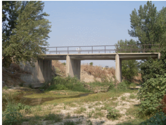
Figure 27: Bridge over the Vega River in Santo Tomé (Jaén), with a Gantry of 3 Spans (6 m +8 m+6 m) and a Reinforced-Concrete Continuous Slab Deck, 1933. Carlos Fernández Casado, Civil Engineer
