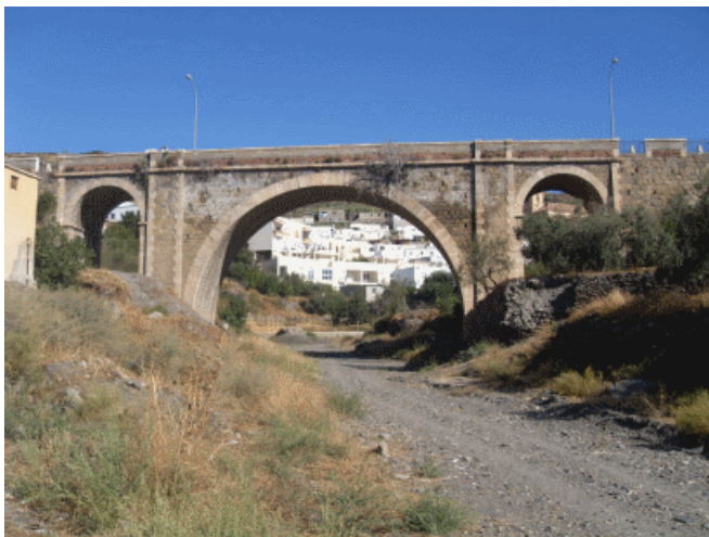
Figure 14: Gérgal Bridge (Almería), with a 20-m-span main Arch and Two 6-m-span Access Arches, on the Primary Road from Las Correderas to Almería. Last Quarter of the 19 th Century
