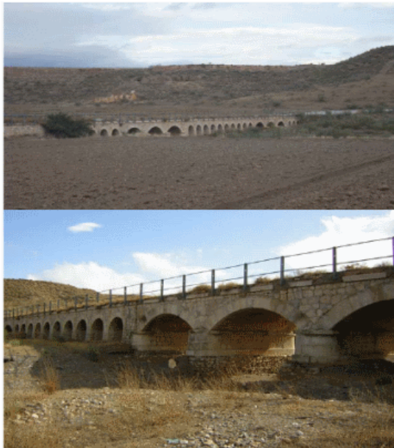
Figure 17: Bridge of Rambla de Valcabra in Caniles (Granada), on the Secondary Road from Baza to Huércal Overa by way of Purchena. Last Quarter of the 19 th Century
