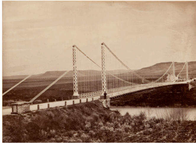
Figure 7: Suspension Bridge of 105 m Span over the Guadalquivir in Mengibar (Jaén), on the road from Bailén to Motril, 1845. Eugenio Barrón, Civil Engineer. Disappeared in 1932. Graphics Archive CEHOPU-CEDEX
