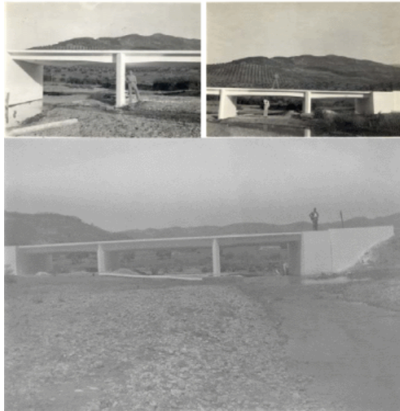
Figure 6: Bridge over the Onsares River, on the Provincial Road from La Puerta de Segura to Siles (Jaén), with a Portal Frame of Three 20-m Spans, 1933. Carlos Fernández Casado, Civil Engineer. Recently Replaced by a Prestressed-concrete bridge. Archive of Carlos Fernández Casado, CEHOPU-CEDEX
