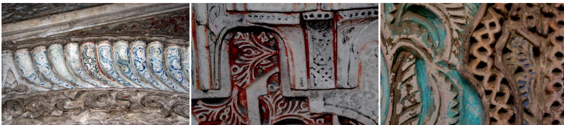
Figure 1: Polychrome residues in medieval plasterwork. Left: Royal Chamber of Santo Domingo, Granada. Center: The oratory in the Madrasa, Granada. Right: Royal Alcazar of Seville.
