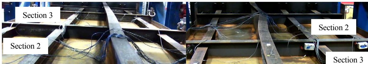
Figure A.7: (Left) Views of the structure at a peak load of 6.59 MN and (right) at a load of 6.25 MN after reaching the peak load.
