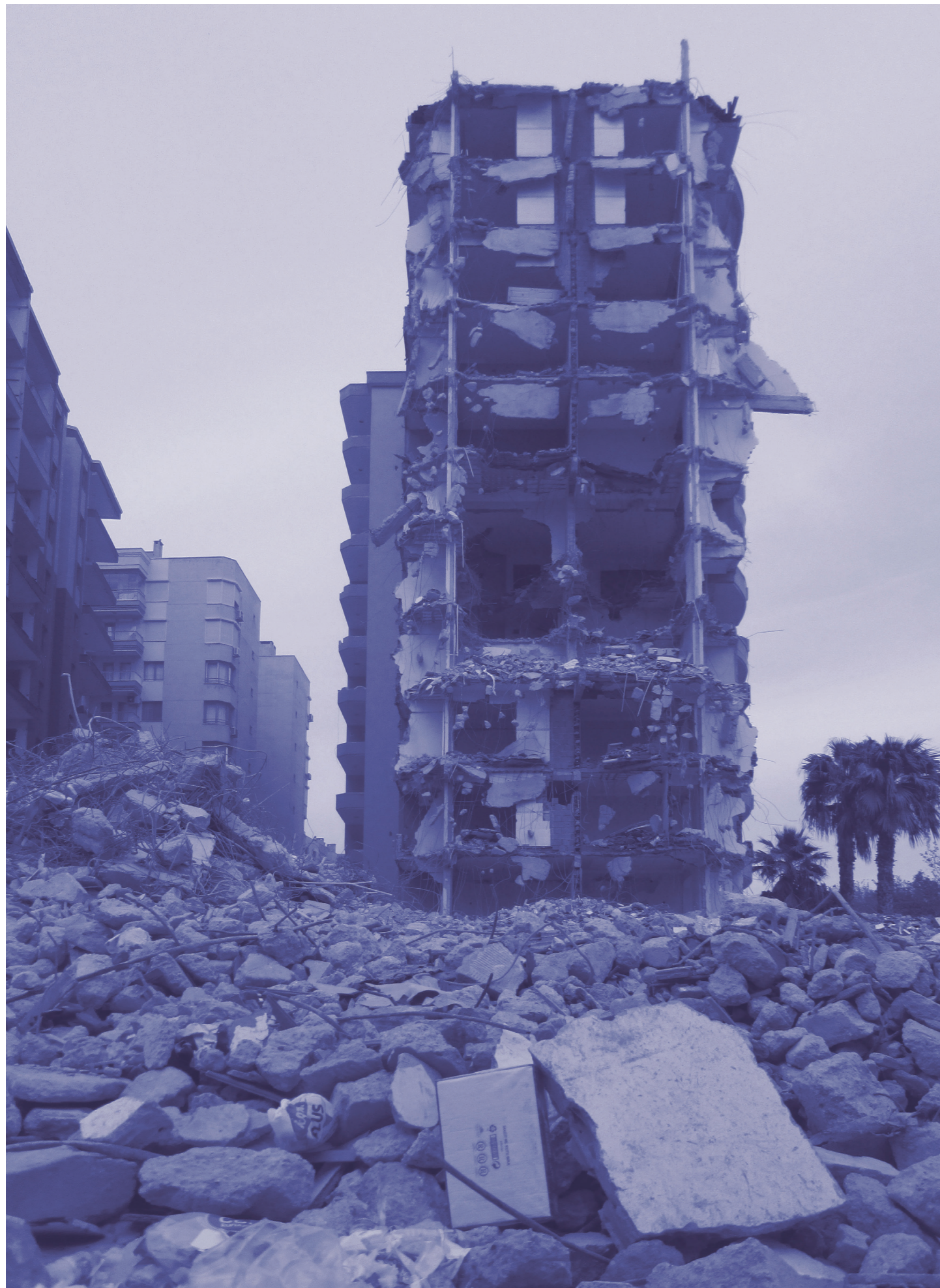
Demolition of buildings in Izmir..
