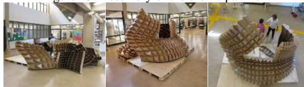
Figure 25: Assembly of the bionic pavilion.
