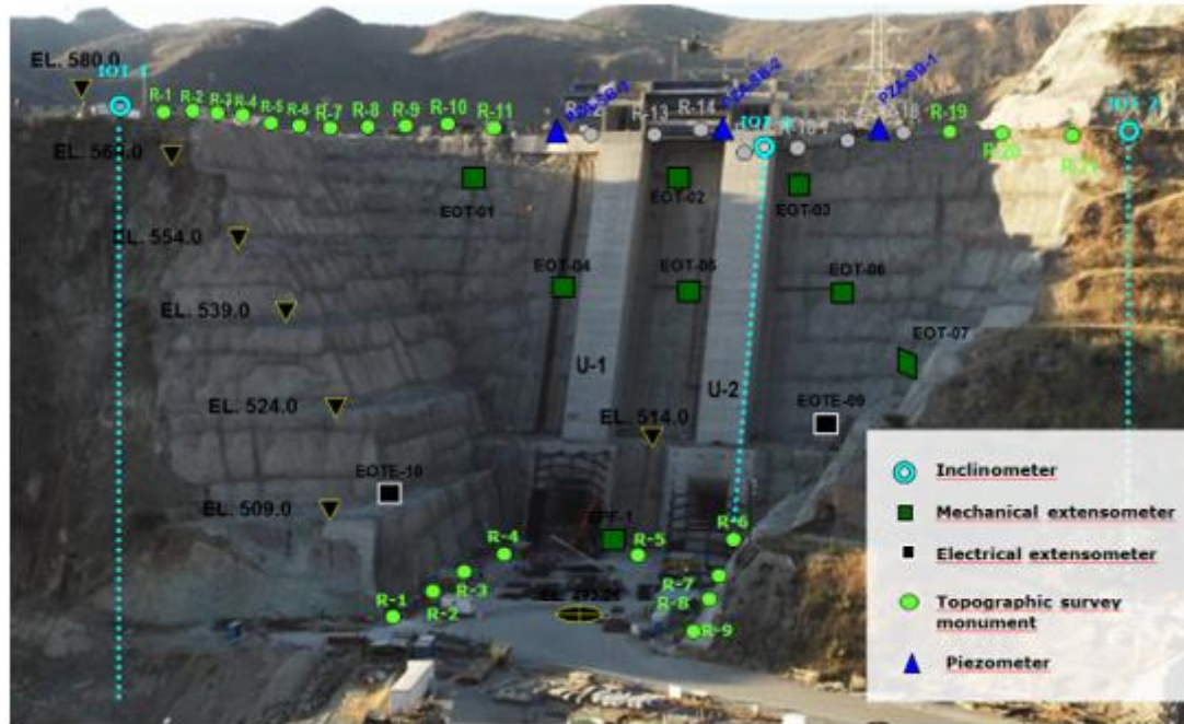
Figure 17. Instrumentation on the slopes of the intake structure
