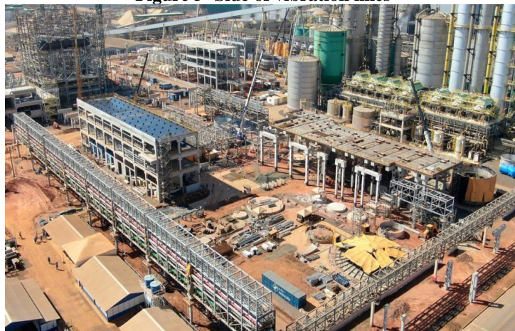
Figure 5- Side of vibration lines
