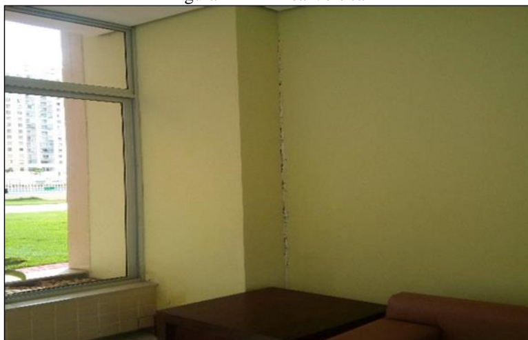
Figura 11 – Trinca Vertical
