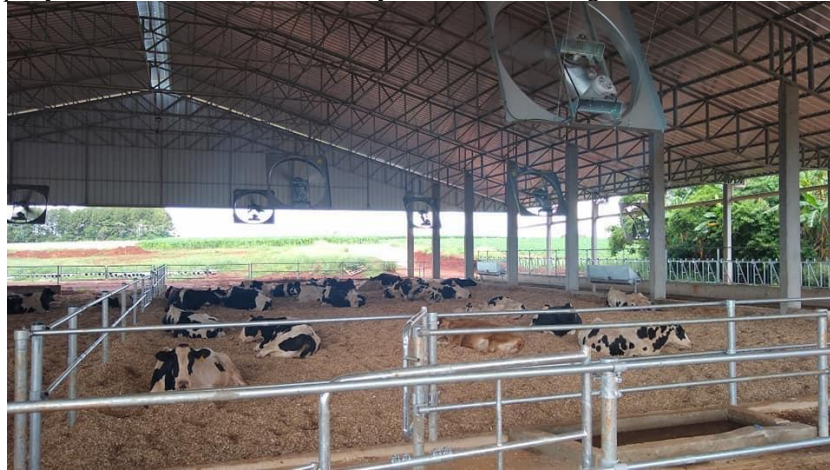
Figure 2. Property with mechanical ventilation system demonstrating the confort of the animals.
