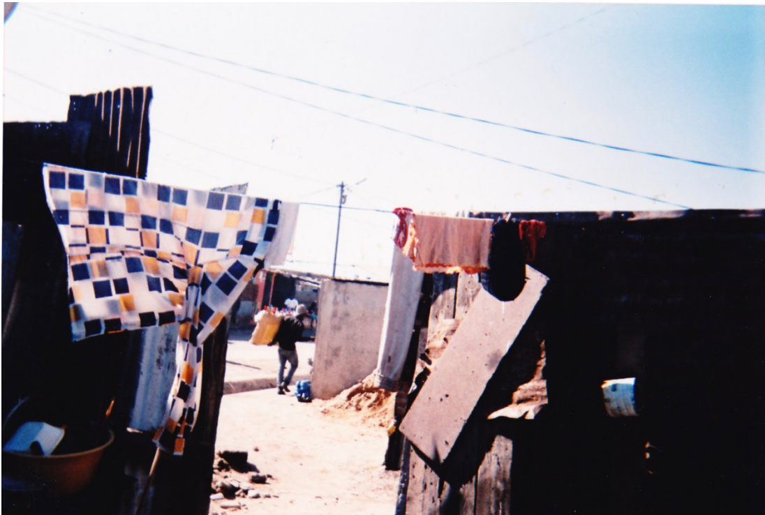
Picture 1: photo taken by José for the « quem sou eu? » project and exhibited at the day centre. José told me that with this photo called «the door of the house, which has fallen down» he wanted to show what he meant by not having privacy with neighbours.
