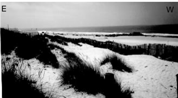
Photos 3 and 4 - Sand traps (fences) installed along the foredune's seaward face dunes
