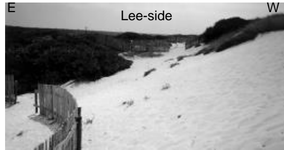
Photo 5 - Installation of fences at the leeside of the dune to promote sand trapping and restrict inland-side access
