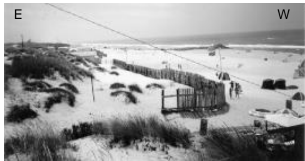
Photos 3 and 4 - Sand traps (fences) installed along the foredune's seaward face dunes
