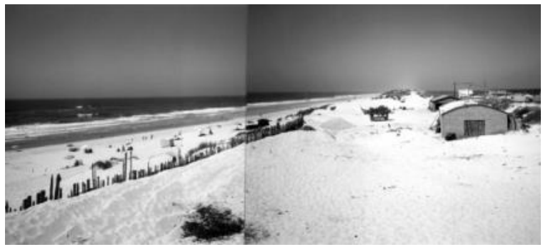
Photo 1 - Dune regeneration induced by the installation of fences (sand traps)
