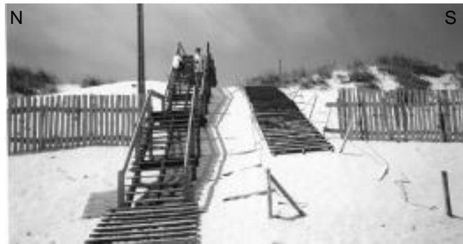
Photo 6 - Elevated walkways built for trampling control
