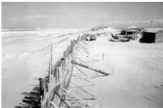
Photo 1 - Dune regeneration induced by the installation of fences (sand traps)
