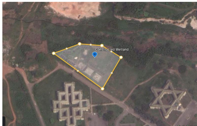
Figure 2: Wastewater treatment facility (constructed wetland) in Covenant University
