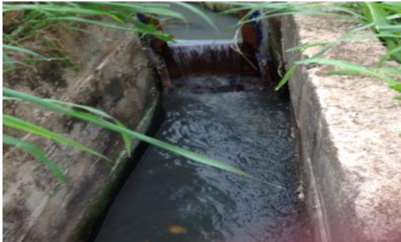
Figure 4: Wastewater Channel and Fabricated weir
