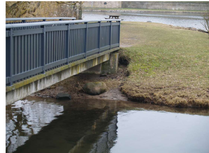
Figure 22: Erosion around bridge foundations. ©Vilborg Thorildsdottir
