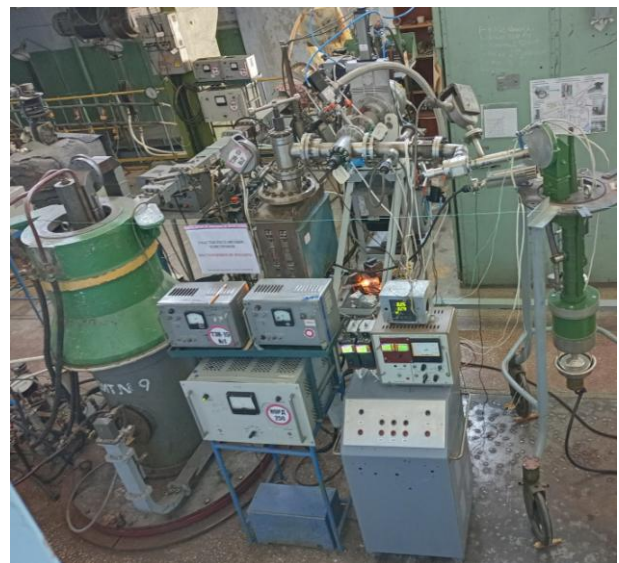
Fig. 3. Configuration of modernized vacuum system during klystron baking and cathode activation
