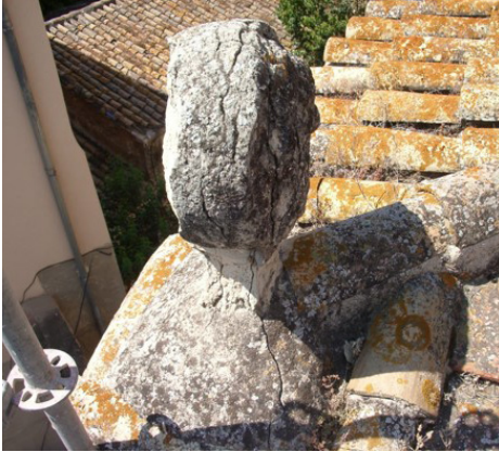
Fisuras y grietas (PF1) Fissures and cracks (PF1)
