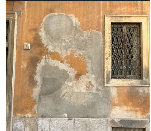
Mortero impropio (RA3) Improper mortar (RA3)
