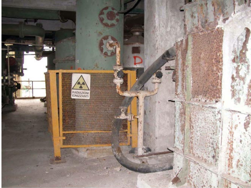
Fig. 9. – Dismissed Phosphate plant. Restricted area due to gamma radiation emission from scales in tanks, mostly, Radium sulphate concretions (ISPRA/ARPA/Eni inspection photo of 2006).
