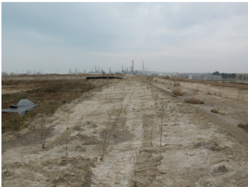
Fig. 7. – Phosphogypsum landfill before complete remediation (ISPRA/ARPA/Eni inspection photo of 2006).
