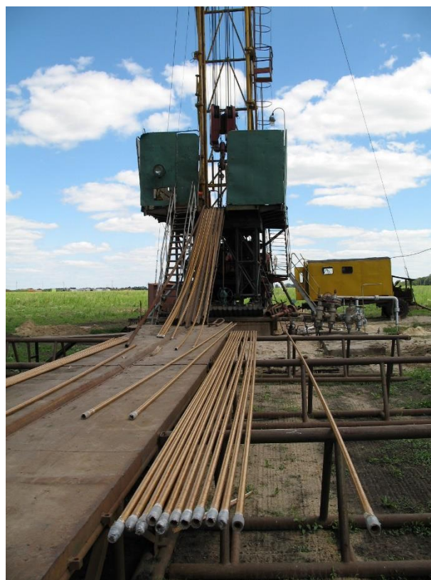
Figure 12: Fiberglass pipes with a diameter of 25 mm for gas well
