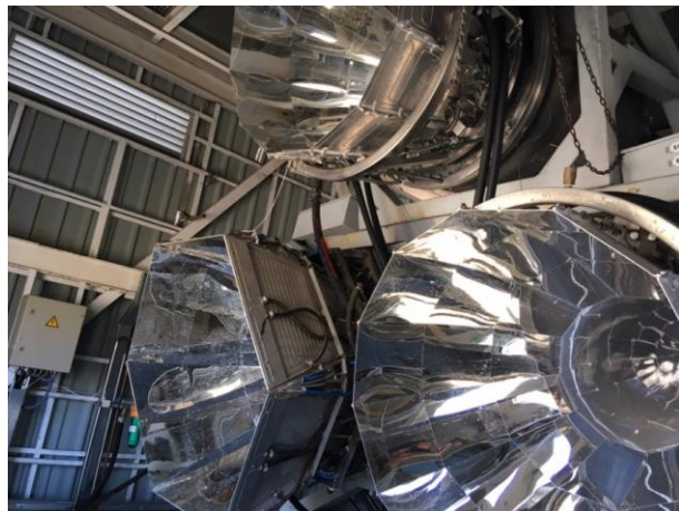
750 kW Hydrosol Plant (3 reactors)
