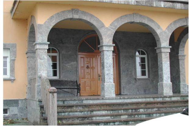
**Figure 1.** Stairs and lintels made of serpentinites from Galicia at the entrance of the town hall of the village of San Ramón de Moeche (A Coruña).
