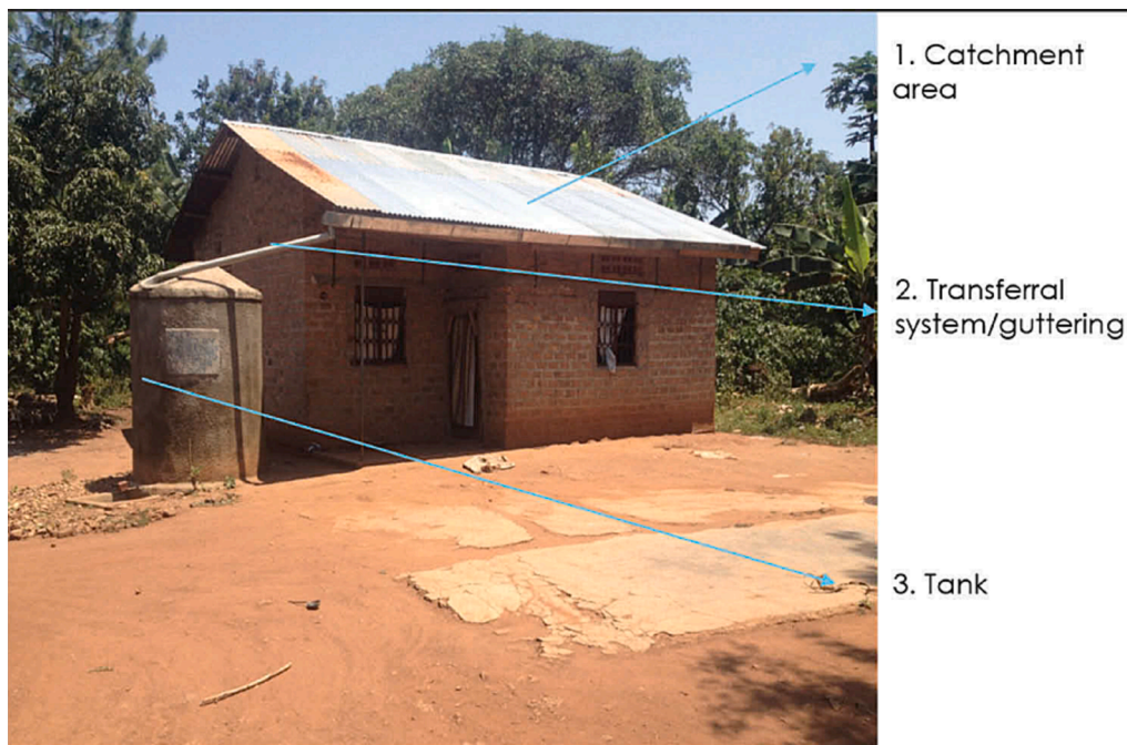
Fig. 5. Schematic indicating basic configuration of domestic rainwater harvesting systems in Uganda. Source: Staddon et al. (2018).
