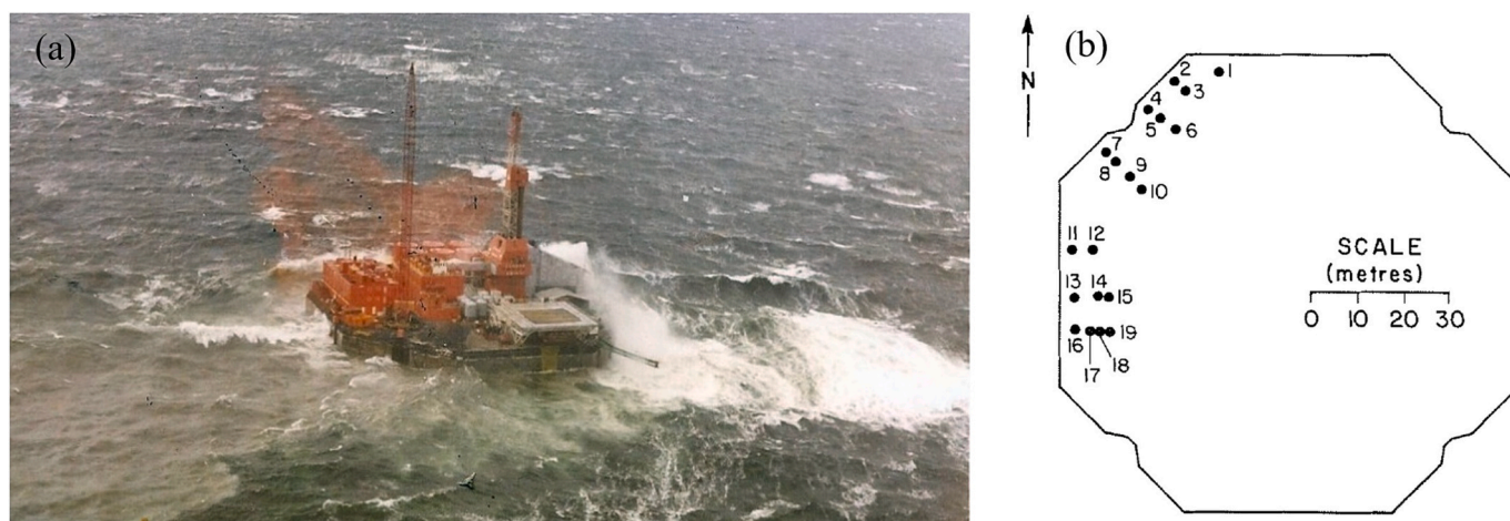
Fig. 2. (a) Tarsiut Island, Beaufort Sea (Picture R. R. Ward). (b) Typical layout of measuring drums (black dots numbered) on the island during the field study (Muzik and Kirby, 1992).
