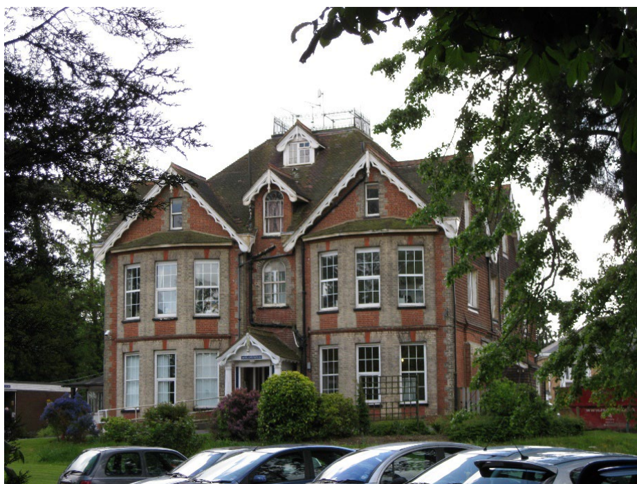
Figure 2. Ifield Park (Photograph 2010. © M G Culshaw)
