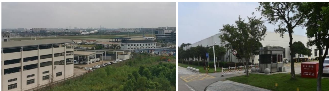
Figure 2. The Ningbo airport and staff restaurant
