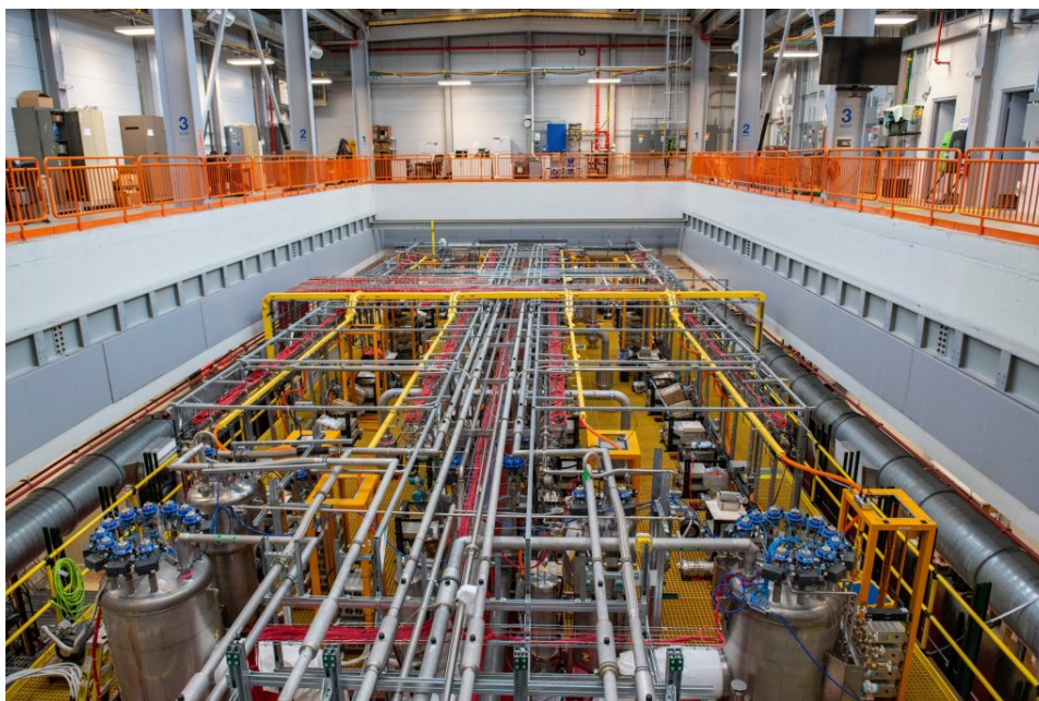
Figure 2.27: Picture of the ICARUS roof at Fermilab during the commissioning phase and before the Top CRT installation.
