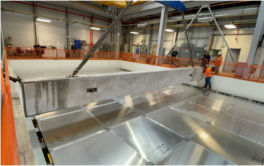
Figure 2.23: Picture taken during the deployment of the first concrete overburden block on top of the ICARUS CRT.
