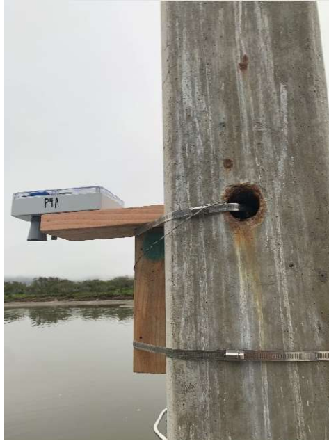
Figure 23: Hose Clamps to secure L-Shaped Platform on Pylon at Morro Bay State Park Marina
