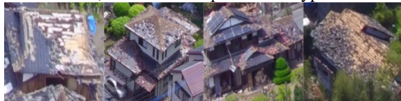
Figure 10. Damage data estimated as collapse in Node. 16.
