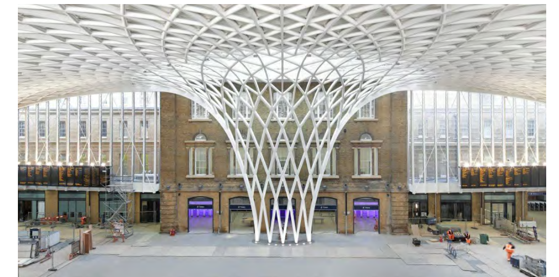
INTERIOR CONCOURSE VIEW
