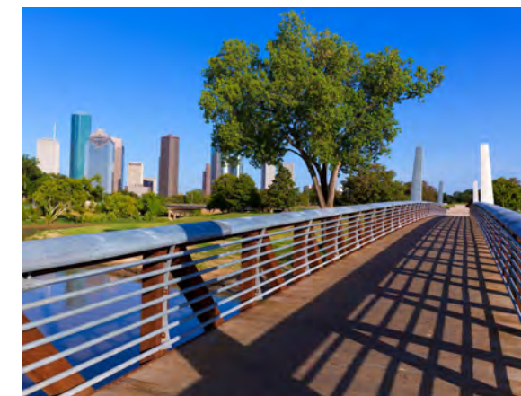
3. BUFFALO BAYOU BRIDGE
