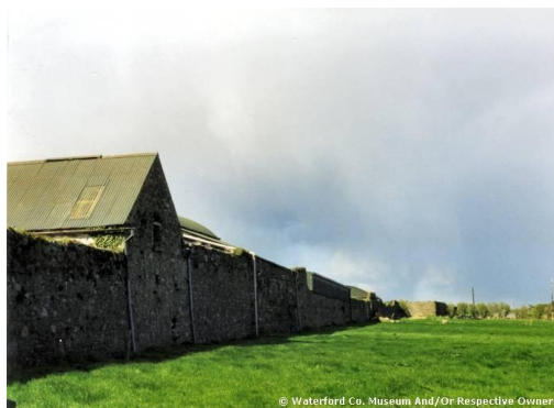
Figure 2.1: Walls At New Geneva Barracks Near Waterford, 1998
