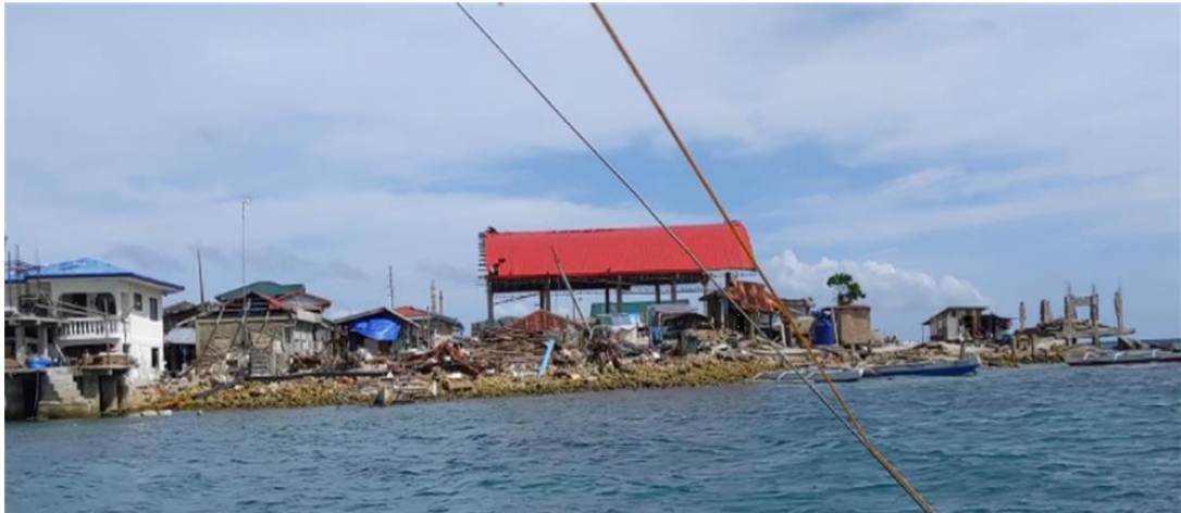
Figure 5. Damaged structures at the coast of Pangapasan Island.
