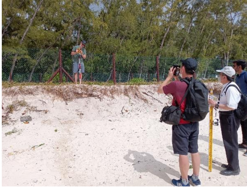
Figure 40. Coastal erosion in Belle Mare, Mauritius.
