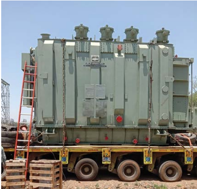
Figure 1. Transformer received loaded on multi-wheeled low-bed trailer
