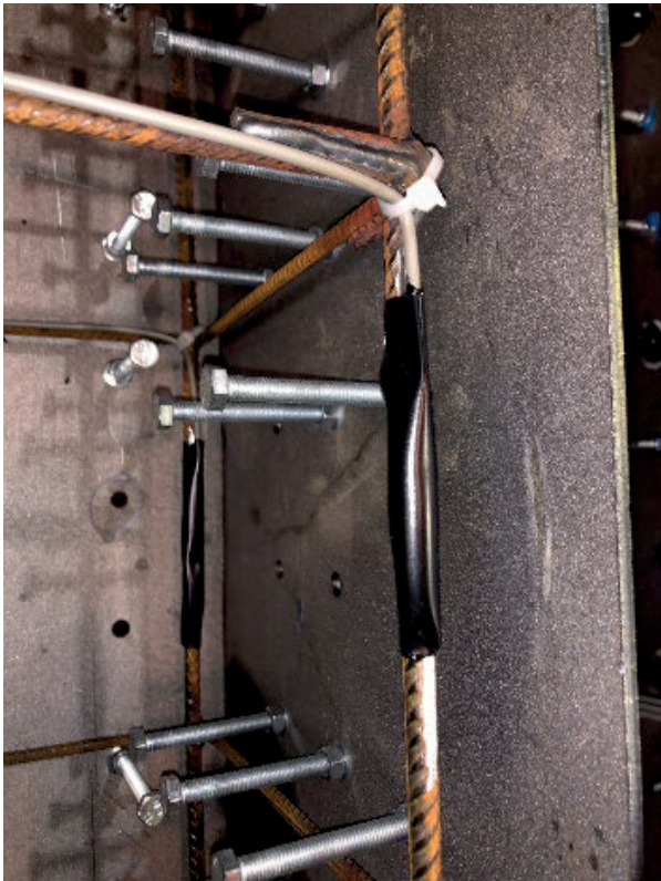
Figure 2. Resistive-strain sensors. Installation and protection
