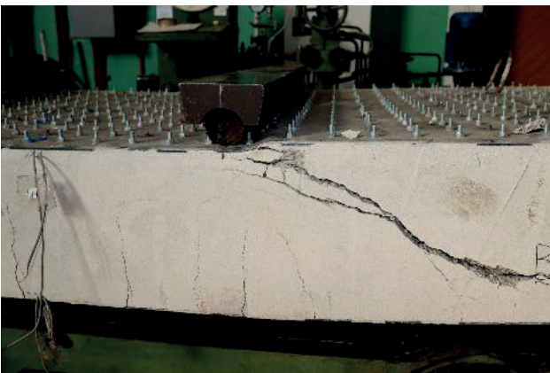
Figure 7b. Typical view of destruction of models tested for bending
