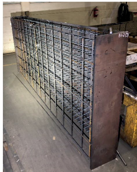
Figure 1. Steel plates and frame reinforcement
