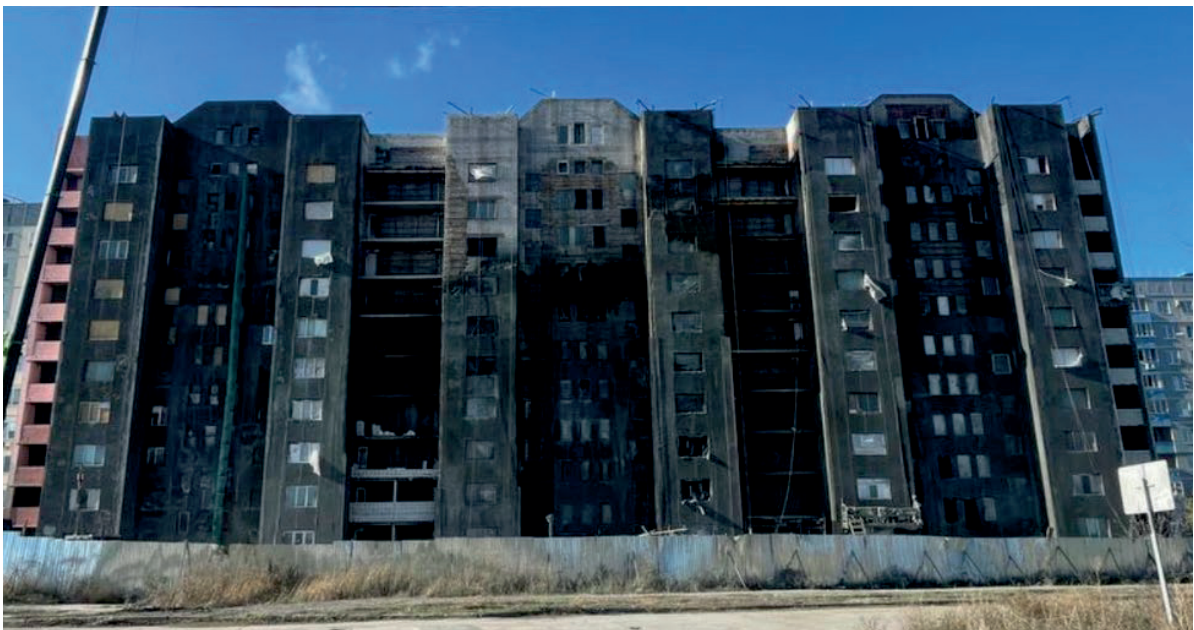
Figure 15. The strengthening of masonry walls of a multi-storey building
