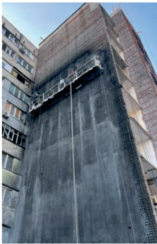
Figure 14. Strengthening masonry walls of a multi-storey building
