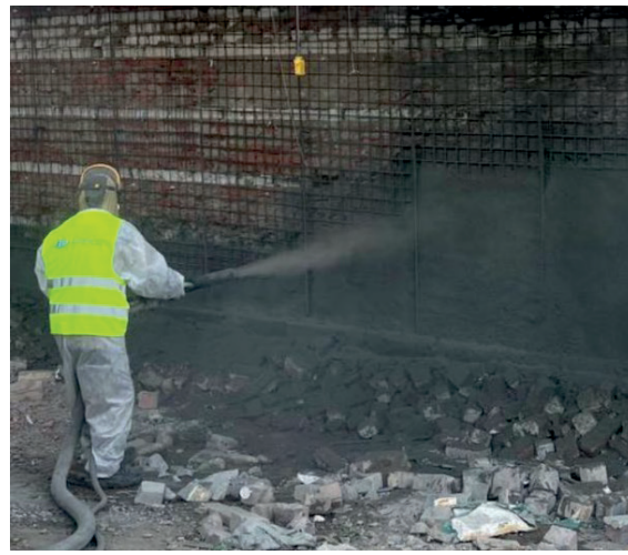
Figure 14. Strengthening masonry walls of a multi-storey building
