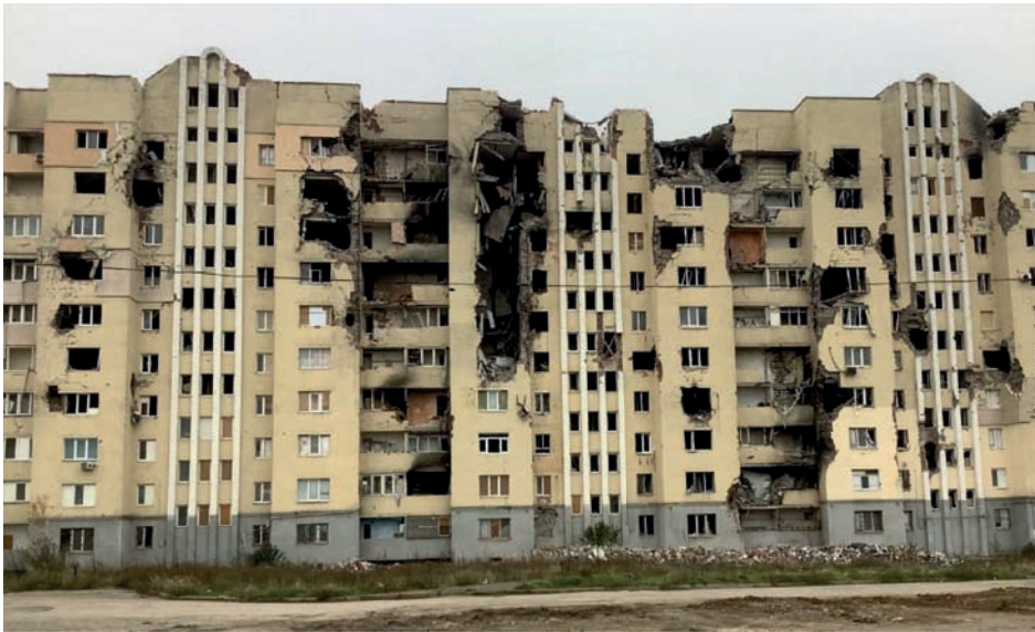
Figure 12. General view of the building described in this paragraph
