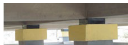
Figure 2. View showing locations of base isolators in the building
