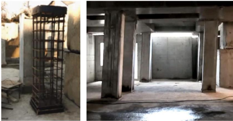
Figure 2-4 Rocking columns in bottom ‘kinematic bearing’ story: (a) completed (left) and unfinished (right) column; and (b) rocking of columns in a free-rocking-motion test (Bachmann et al., 2017).
