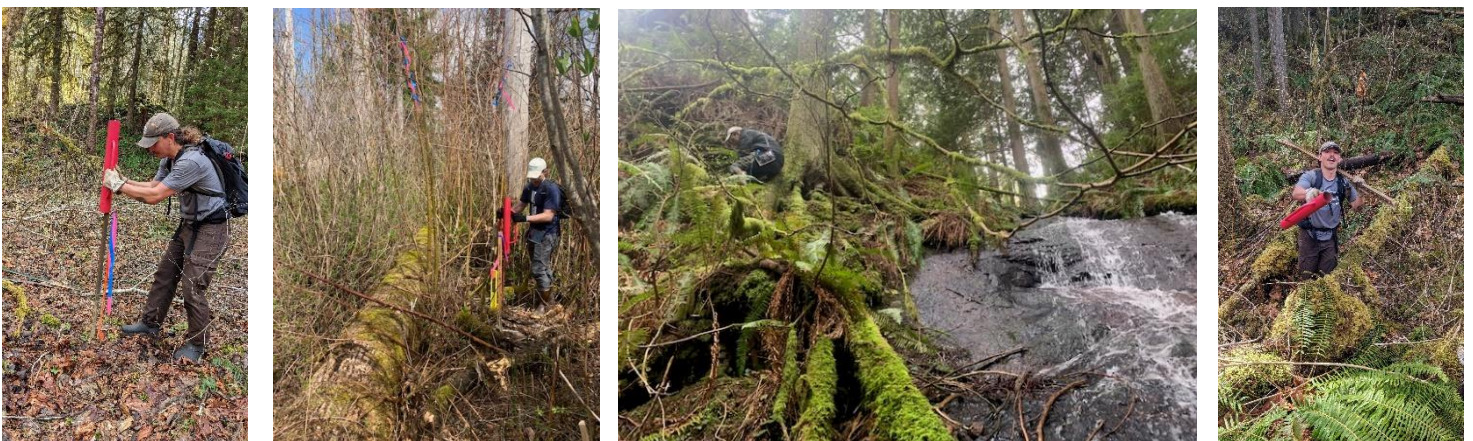
Figure 7: Adriano (far left) and Bryce (mid-left) pounding T-posts in at surveyed points for easier locating in the future. (Mid-right) Bryce searching for a long-lost survey monument on the hillside among tree roots. (Far right) Adriano carrying T-posts and pounder through thick brush along property border. (de Oliveira & Auburn)
