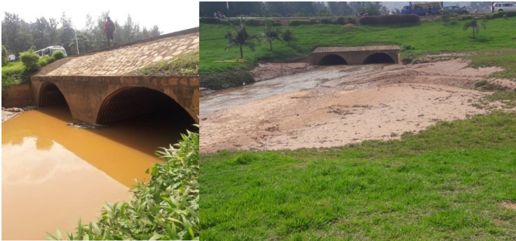
Figure 1: Existing culverts under the road Nyabugogo-Muhima-Kacyiru
