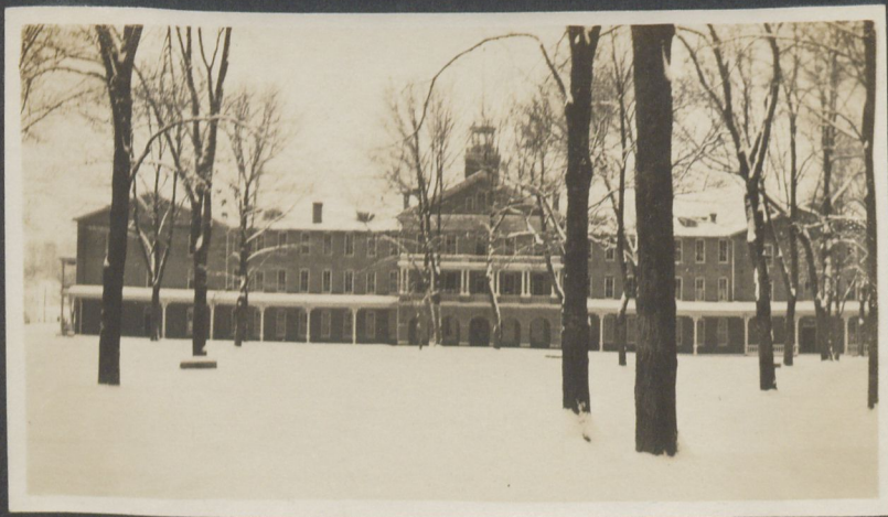
West Building - Hollins
