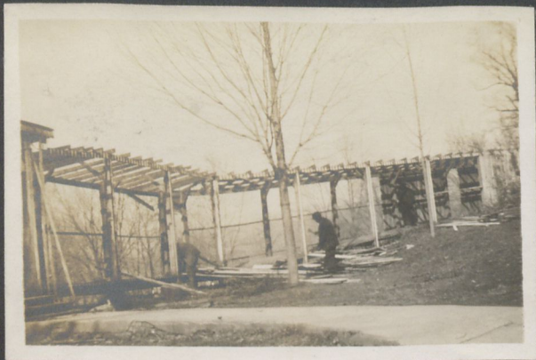
The demolition of the covered way. (Main to Music Hall)
