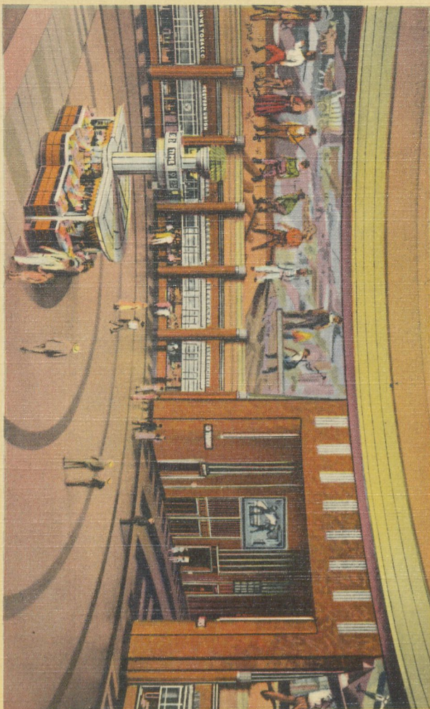
18—Lobby, Union Terminal, Cincinnati, Ohio
