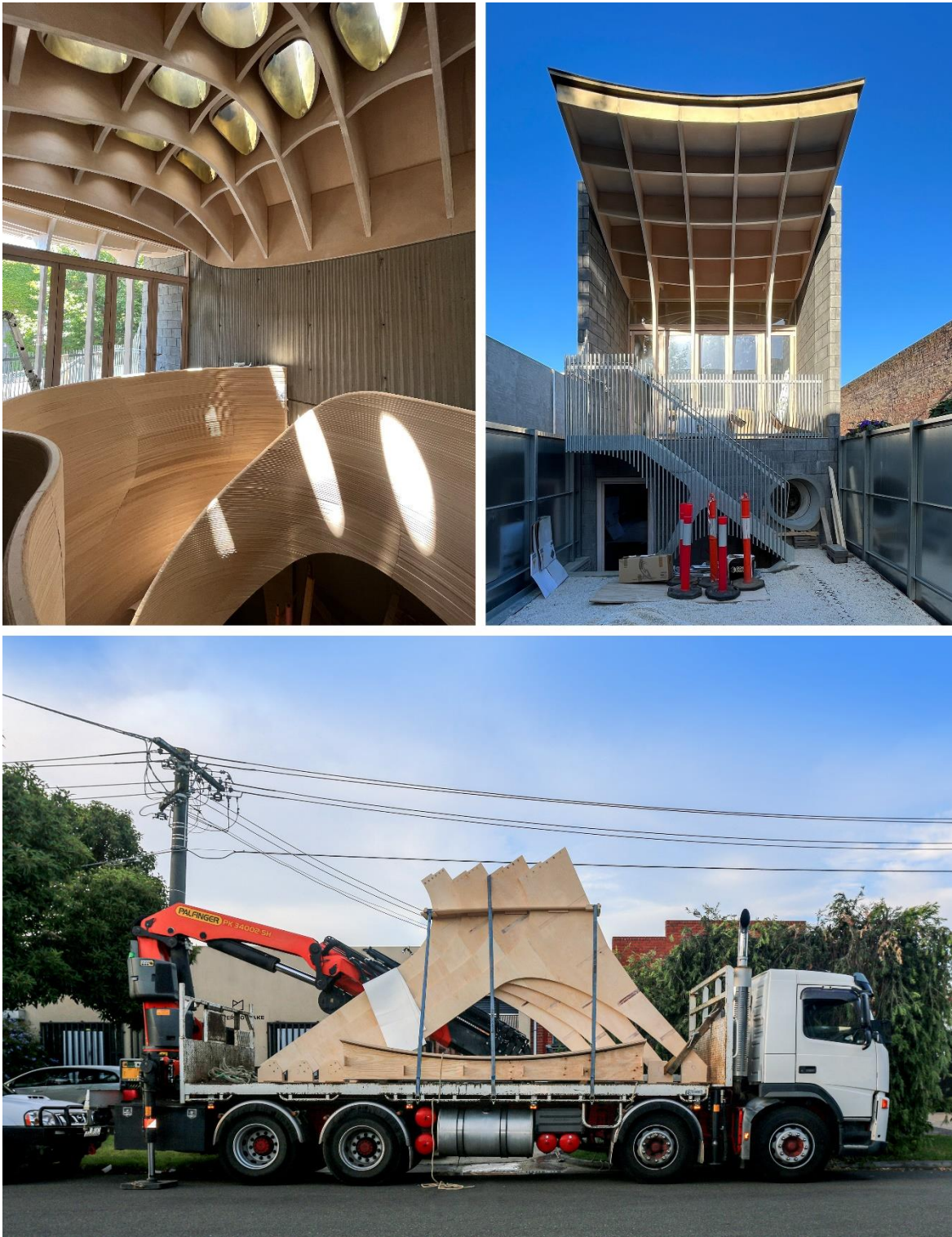
Figure 1. Top Left, the roof's soffit with skylights supported by the concrete boundary wall. Top Right, front elevation of the house with a cantilevered roof. Bottom, urban manufacturing facility of Power to Make. Image showing the loading of CLP roof rafters ready for site delivery.
