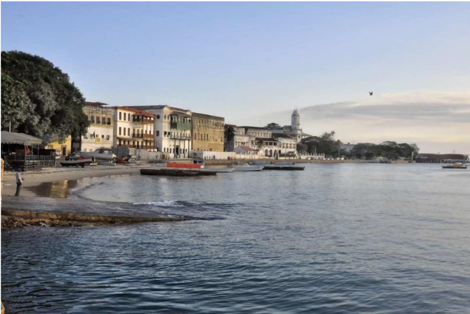
Figure 2. Zanzibar Stone Town waterfront in 2013. Of the buildings and sites visible in this image, several have been part of major restoration projects including Forodhani Gardens, the House of Wonders and the Palace Museum. The former Customs House in the British colonial era (the balconied building to the left) was restored and transformed into a hotel in 2014. Wikimedia Commons: https://en.wikipedia.org/wiki/File:Stone_Town_Waterfront,_Zanzibar_%2810163203685%29.jpg .
