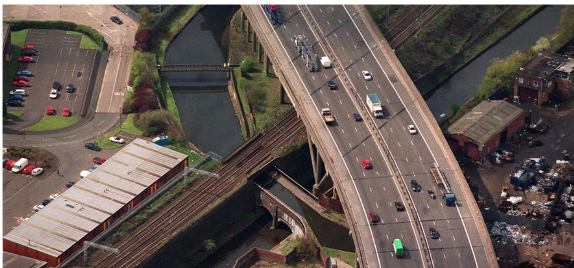
Aerial view of the M5 motorway crossing New Main Line canal in Sandwell with the Stewart Aqueduct and railway lines.
