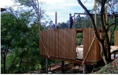
FIGURA 95 - MONTAGEM DOS PAINÉIS (VILA TAGUAÍ).
