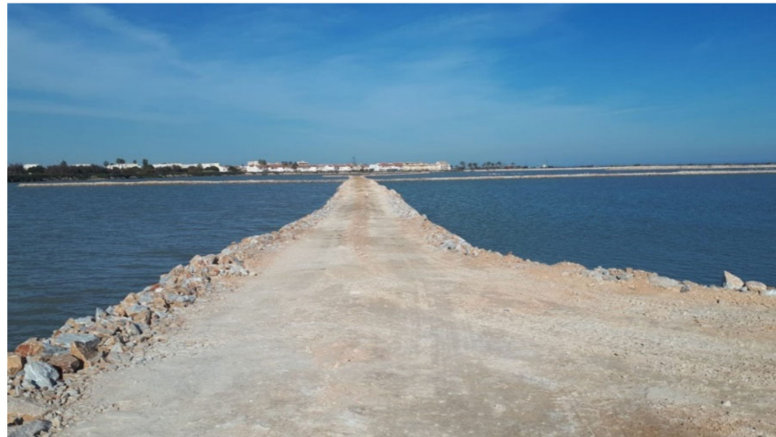
Figure 7. New sandy dikes separating salt ponds (Source: LIFE-SALINAS Project).
